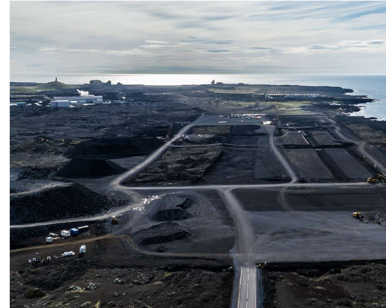
Construction of Samherji's aquaculture facility by Reykjanes Power Plant.
