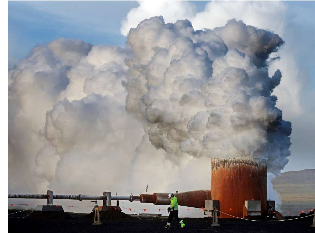
Borehole at Eldvörp tested.
